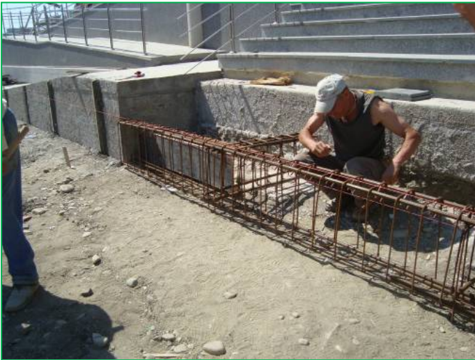
Corp C – Armare trepte intrare
