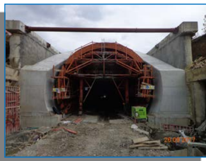
Tunel Daneş - Betonare tunel artificial
